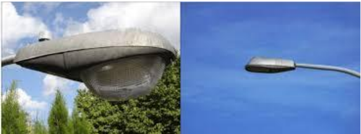
Cobra Head lights - Drop Lens on the left; Flat Lens on the right.
